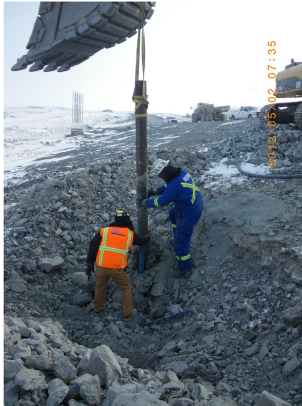
Photo 1: Excavation and removal of 6" steel pipe from around ND-IN-120-3
