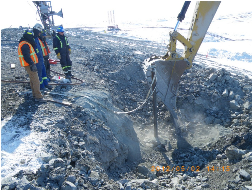
Photo 3: Back-filling of ND-IN-120-3 in lifts of core material and ROQ.
