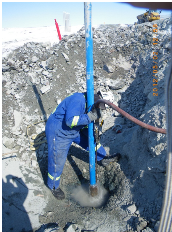
Photo 2: Water lance used to flush material from between the 4" steel pipe and the Inclinator Casing.
