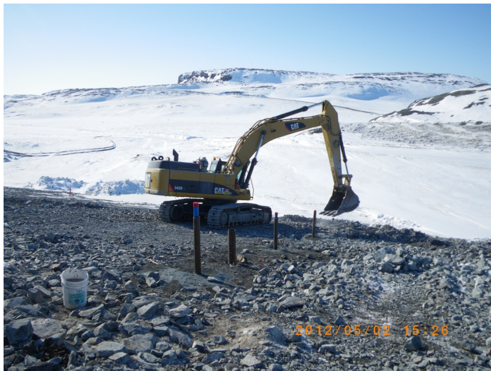
Photo 5: All instrumentation along Station 1+20 installed. The 4" Sched 40 Steel Pipe still to be installed in ND-DSP-120 and the top caps fabricated and installed on all instrumentation.
