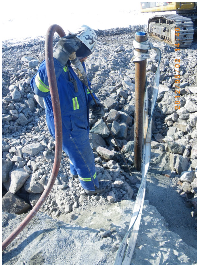
Photo 4: The water lance was used to saturate the core material around the Inclinator Casing and 4" steel pipe.
